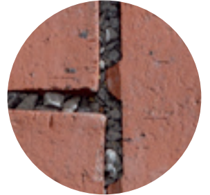
Joint drainant de 6 mm = part des joints: 10%
