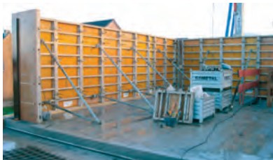
finishing concrete, precise work
