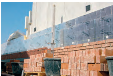
Ground slab polyurethane insulation
