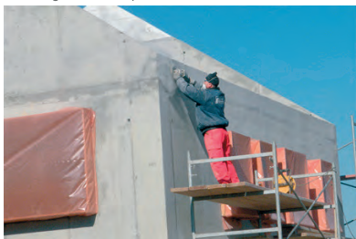
Insulation PUR, 20 to 25 cm thick
