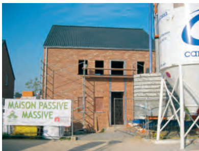
Preparation of formwork
